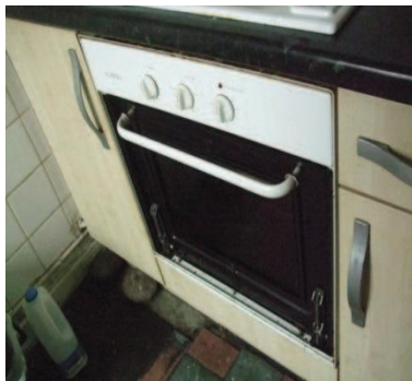
Front panel missing off oven
